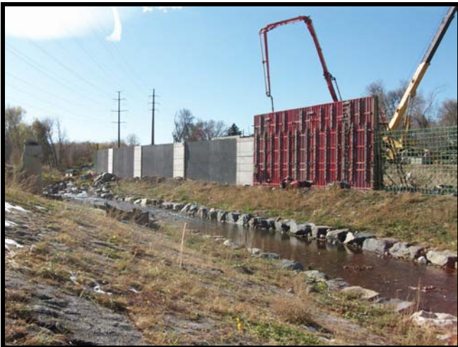
Dry Gulch Retaining Walls- November 2009
