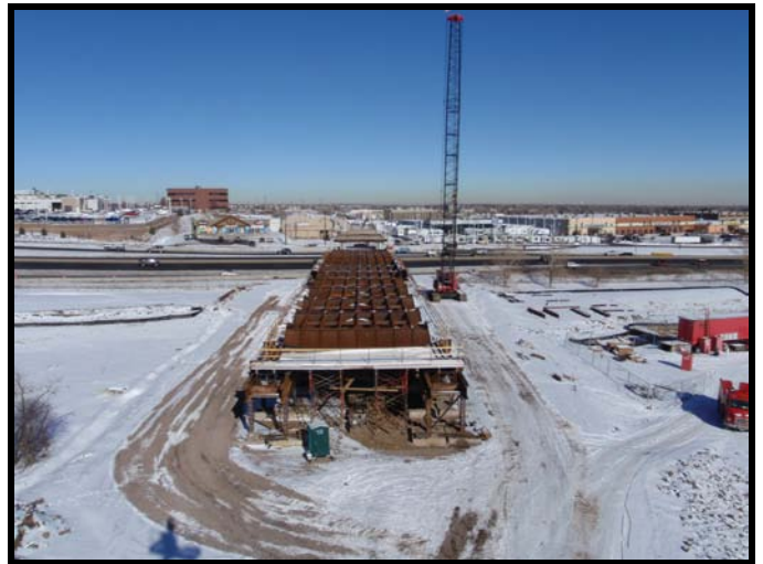
6 th Avenue Bridge (east of Simms/Union)- December 2009
