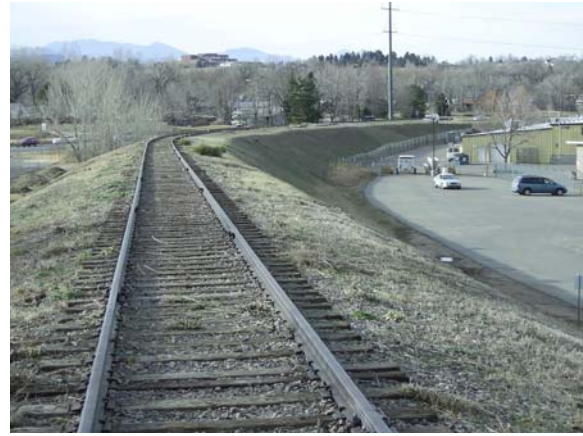
The "Berm" – steep slope
