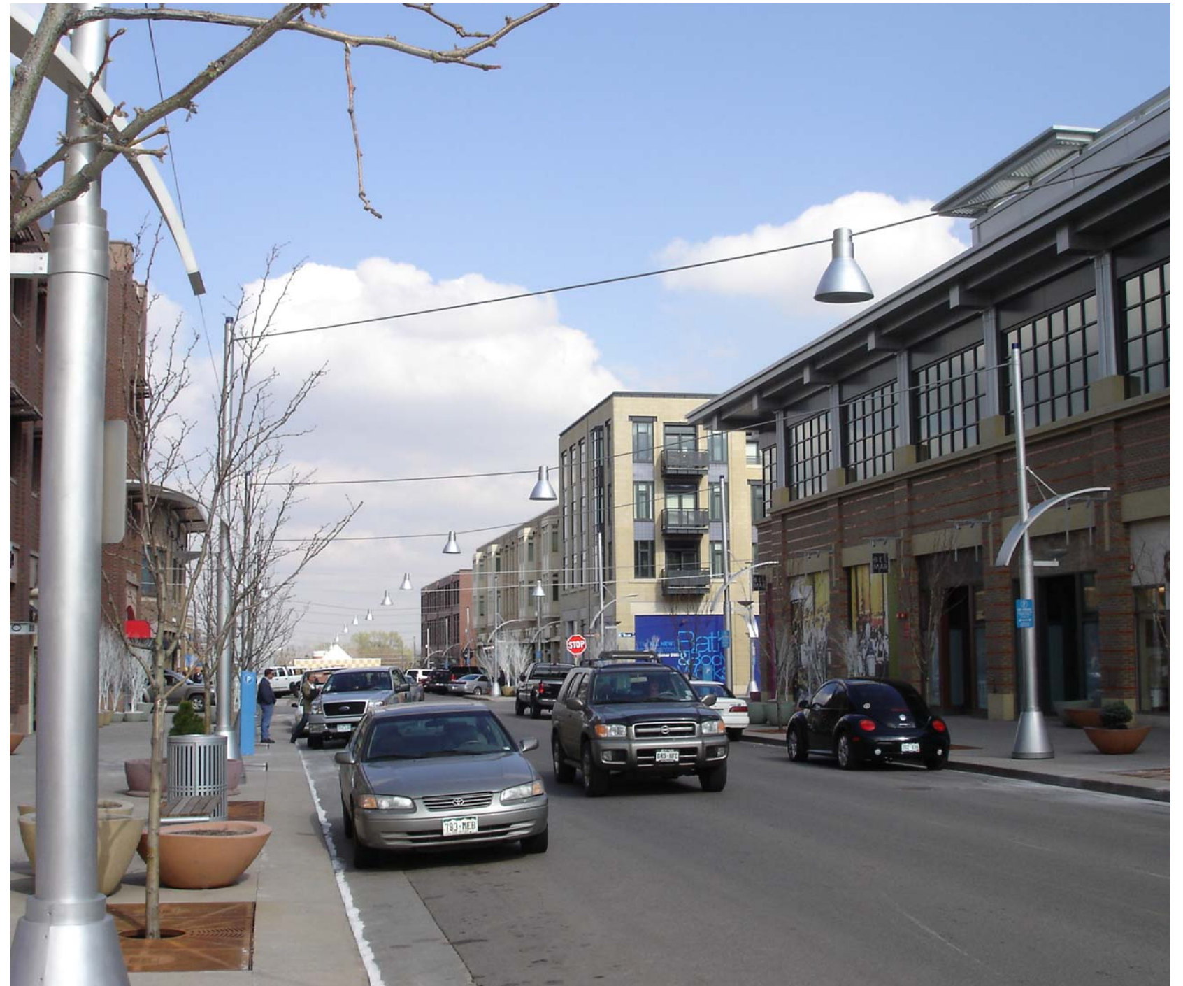
CABLE SUSPENDED LIGHT FIXTURES IN BELMAR
