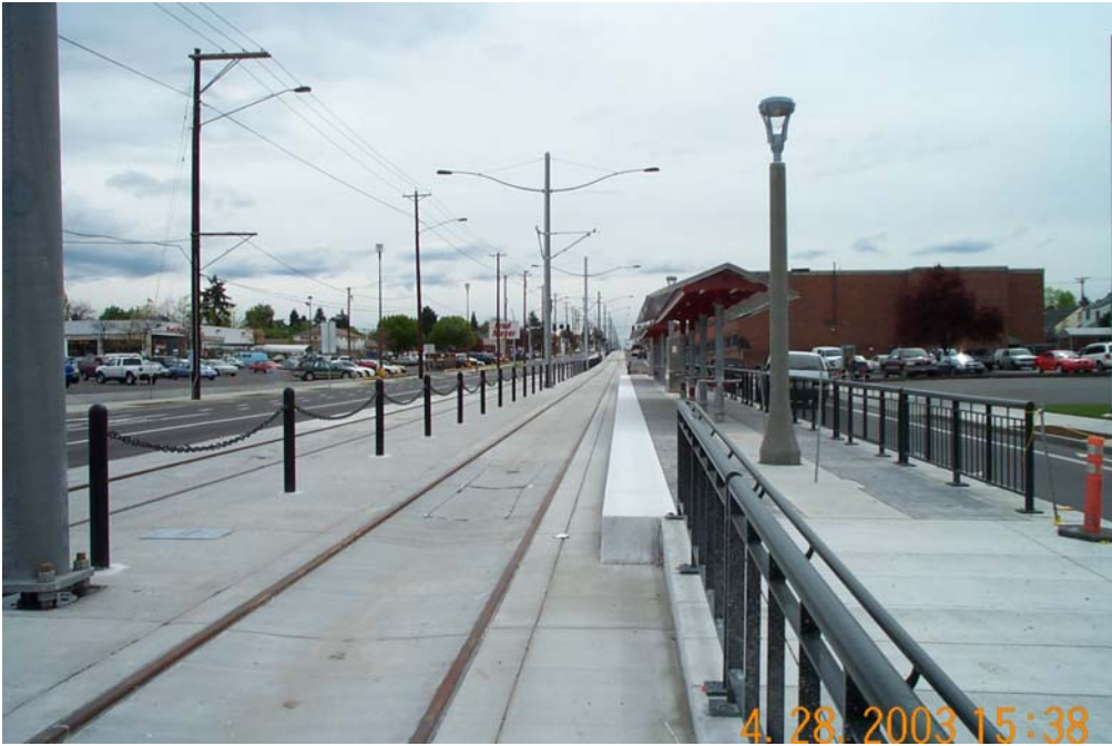
Portland Tri-Met, bollard and chain barrier on Interstate Max
