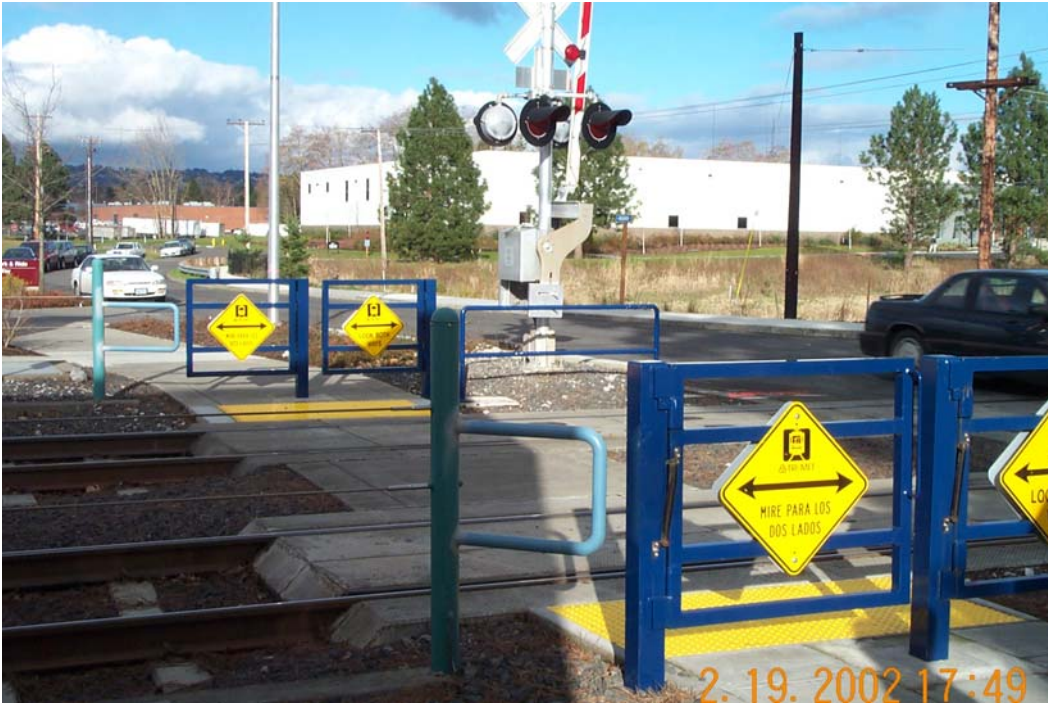
Portland Tri-Met, additional photos showing cable fencing, swing gates and railing
