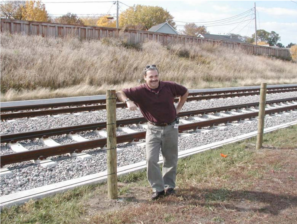
Minneapolis/St. Paul Metro Transit, 4-cable wooden post fence
