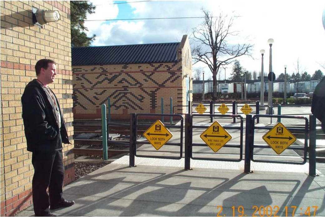
Portland Tri-Met, pedestrian railing, cables and swing gates
