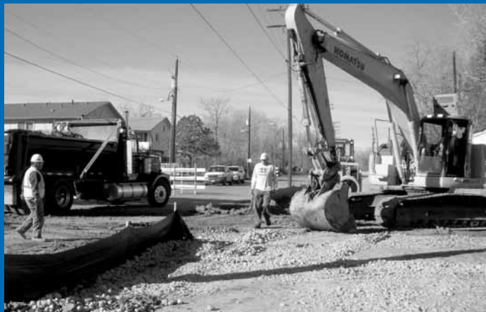
West Corridor crews work on 13th Avenue utility relocation.
