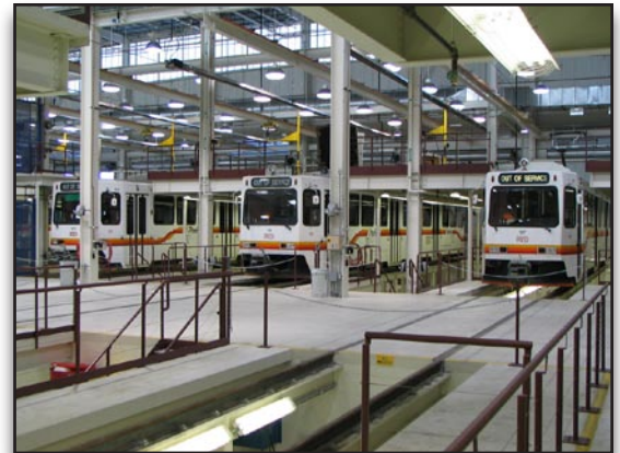
Interior of existing rail maintenance facility
